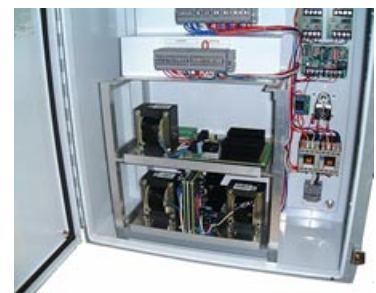
Interior View Of Gate Control Unit (Power Supply): Individual Sector Controls May Be Removed For Servicing Without Touching A Wire
